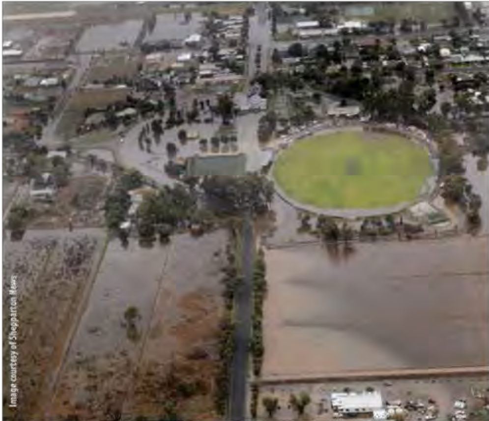
Aerial view of flooding at Katandra West in March 2012 (source: Katandra West Local Flood Guide, December 2016)
